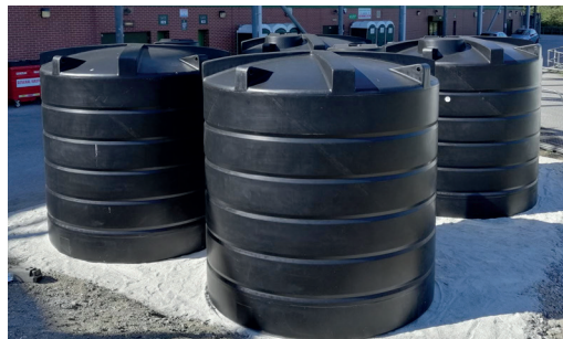
Images: Stand (left); Rainwater harvesting tanks (centre); Rainwater distribution pipe (right).
