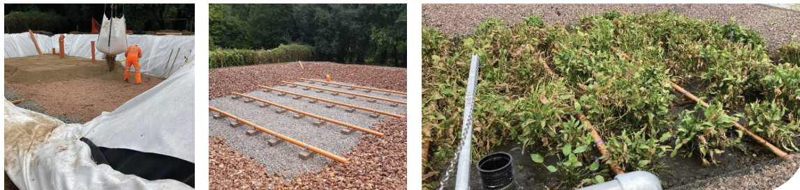
Photographs of the ARMPhos™ system during construction and before and after operation.
