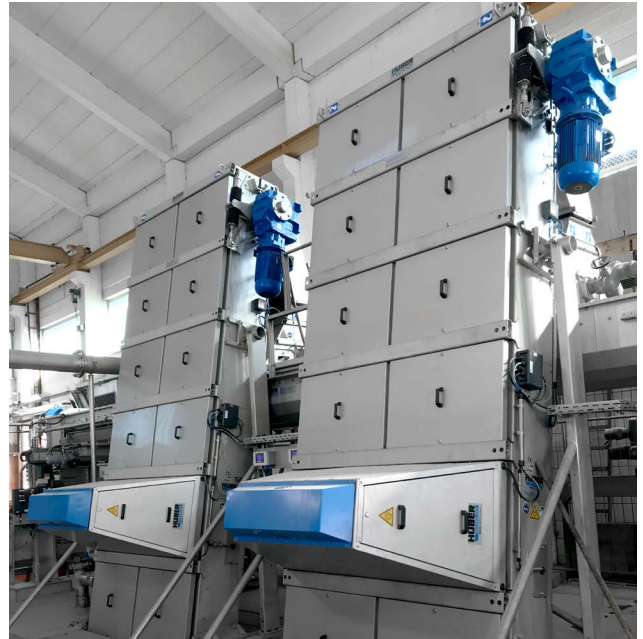
Two HUBER Multi-Rake Bar Screen RakeMax® units equipped with the HUBER Detection System Safety Vision. By detecting critical screenings, Safety Vision prevents damage to the screen and downstream machinery.
