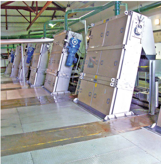
Universally applicable RakeMax® screen for big channel widths and big discharge heights.
