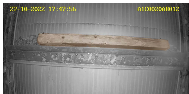
Exemplary images for operator notification – pipe sealing cushion (left) and squared timber (right) on the rake bar of a HUBER Multi-Rake Bar Screen RakeMax®.
