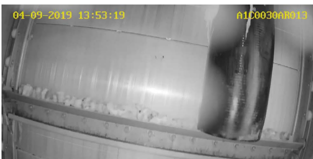
Exemplary images for operator notification – pipe sealing cushion (left) and squared timber (right) on the rake bar of a HUBER Multi-Rake Bar Screen RakeMax®.
