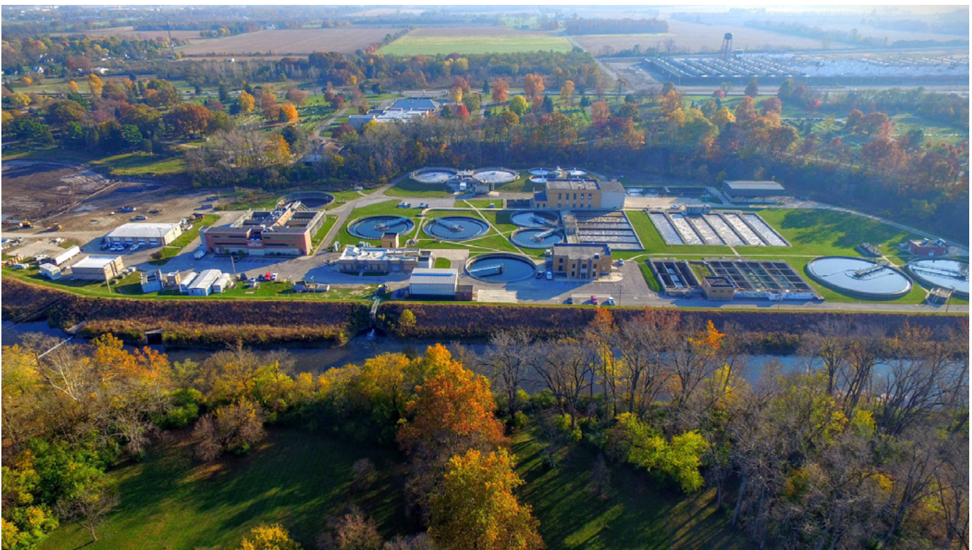
Muncie, Indiana, Water Pollution Control Facility
