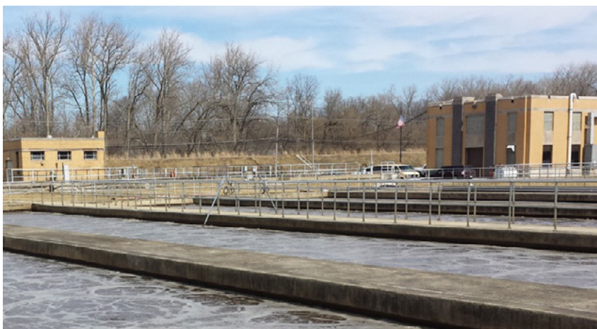
Muncie, Indiana, Water Pollution Control Facility
