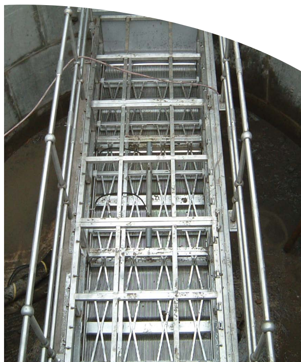
Double sided weir installation
