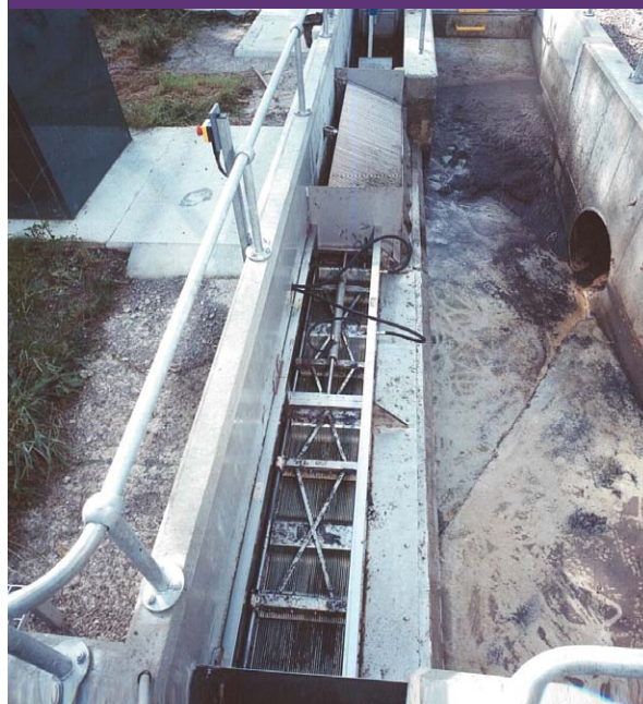
Single sided weir installation
