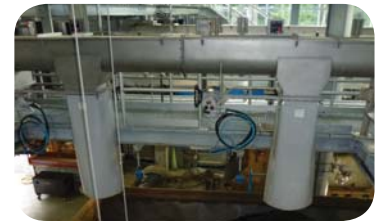
Truck outloading system
