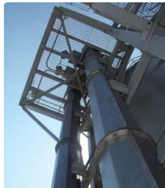
Typical two stage vertical lift sludge conveyors feeding a storage silo
