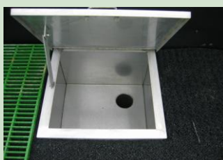
Stainless steel washout box set into surface of media adjacent to access doorway.
