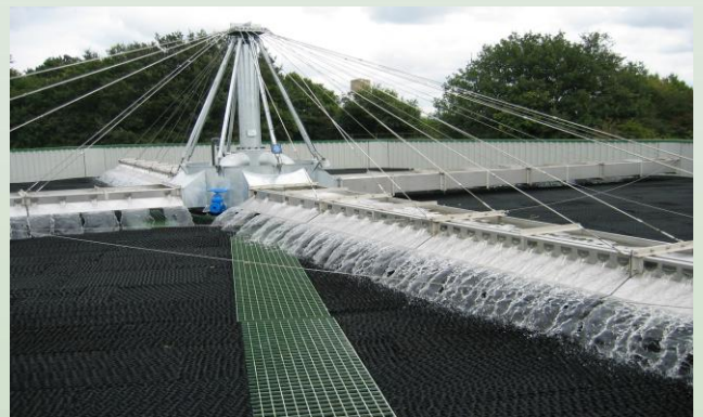
4 Arm motor driven HYCOVER trough arm distributor applying some 360 lt/sec to 20.0 mt dia HYRATE nitrifying filter.
