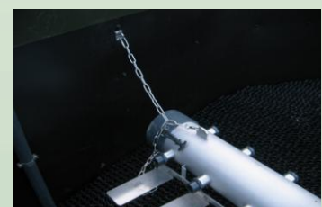
Distributor arms are fitted with Quick strip full flow washout end cap & stainless steel chain..
