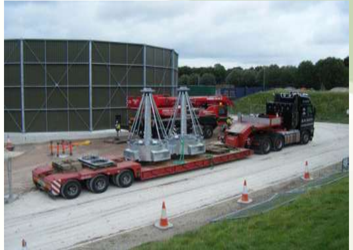
Delivery of HYCOVER Centre Columns.
