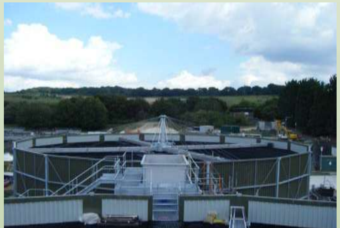
HYCOVER Distributors safely installed.
