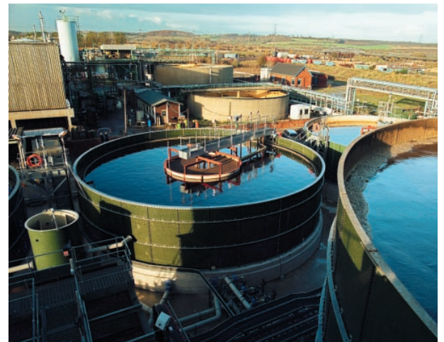
Vitox biological plant at Hickson and Welch
