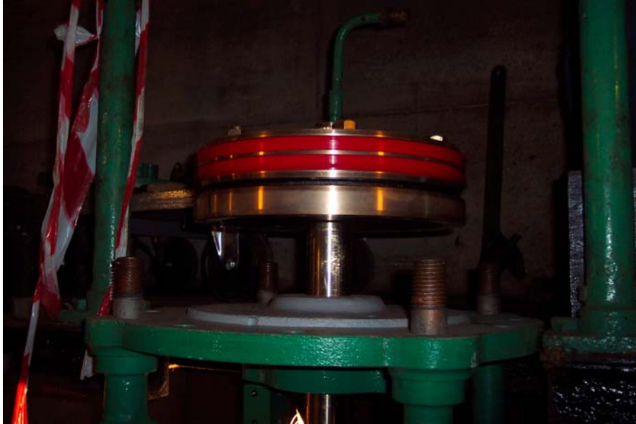
Piston assembled onto the new valve stem
