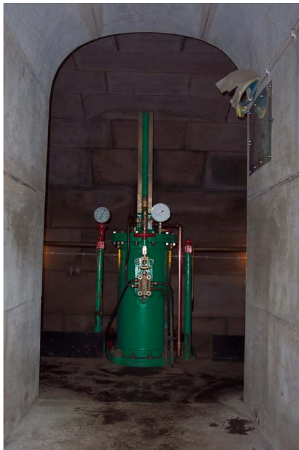
Repainted actuator Howden West
