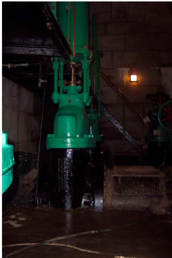
Completed valve at Derwent West
