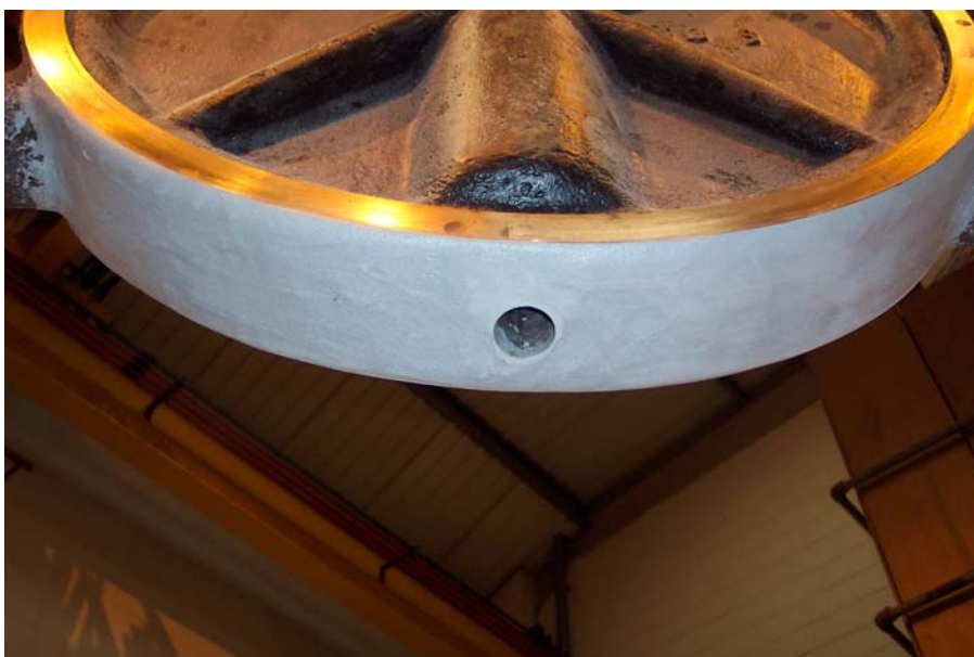
Cavitation repairs Derwent Wedge
