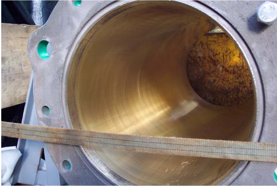
Honed actuator cylinder bore
