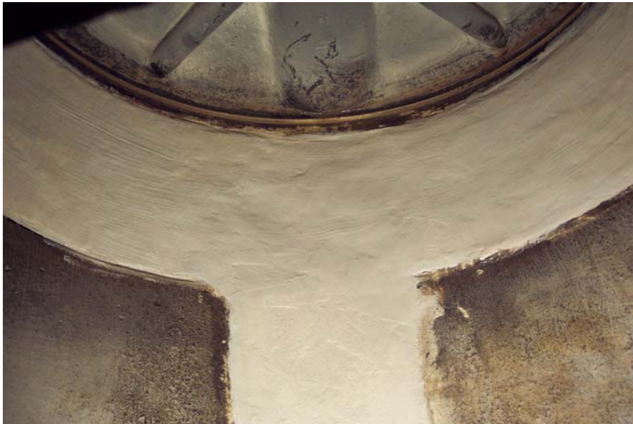
Outlet bore cavitation repairs Howden West
