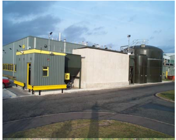
250m 3 /day Discharge to sewer
