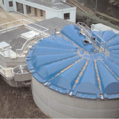
Biological sludge thickening, municipal plant
