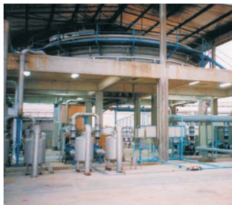
Potable water installation
