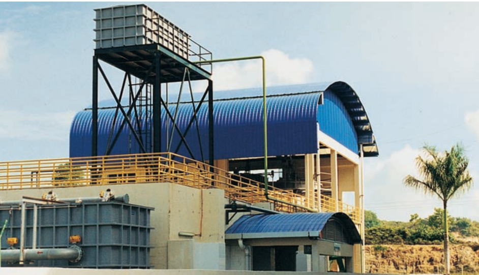
Effluent treatment and water recycling project, rubber manufacture
