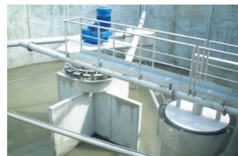
Surface aerator showing floats
