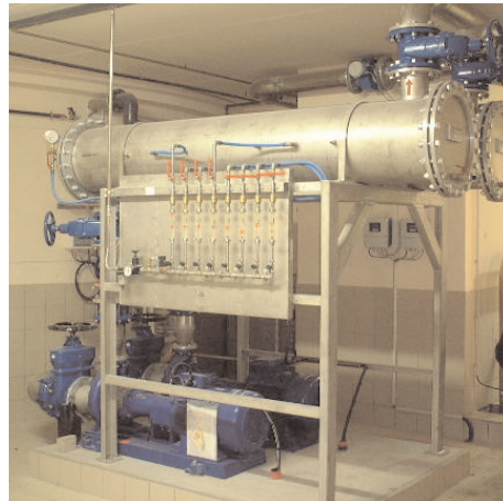
Pressurisation, ADT installation
