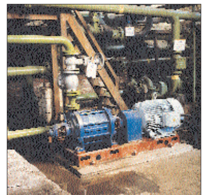
This five stage multi-stage pump is used for pumping water to a hill top reservoir for British Steel
