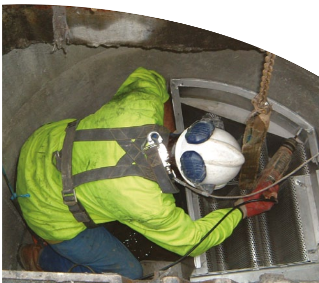
Retro-fit installation of screen.
