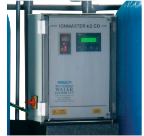
Facia mounted message display provides user information
